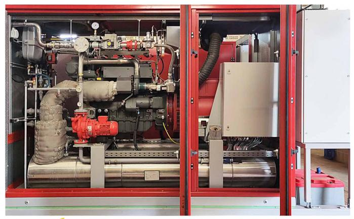
BK<sup>3</sup> builds CHP modules for common fuels and also offers solutions for special applications such as associated petroleum gas or landfill gas. Essentially a CHP consists of a motor (center right), which is usually gas powered, generating electricity andt emitting heat at the same time. Heat exchangers (bottom left) then use this waste heat to heat rooms or process water. The control unit (far right) controls operation.
