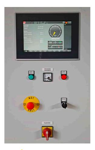
The control unit controls operation of the CHP. After the migration, BK<sup>3</sup> introduced a touch panel for this purpose.
