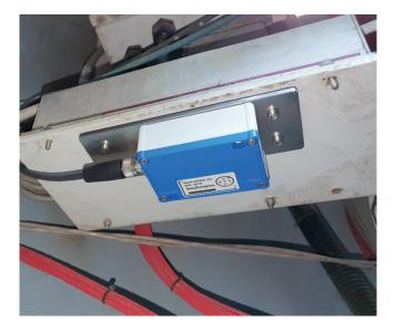
A cost-effective 2D MEMS acceleration sensor provides the vibration data in the most basic configuration. Furthermore, the use of additional sensors, which can be positioned at different levels within the load-bearing structure (tower, transition piece, and foundation), enables an even more detailed evaluation.
